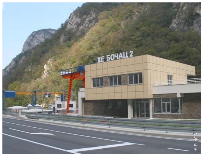
Bocac II, Bosnia-Herzegovina
