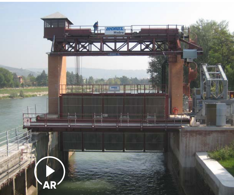
Chievo Dam, Adige River, Verona, five StrafloMatrix units
