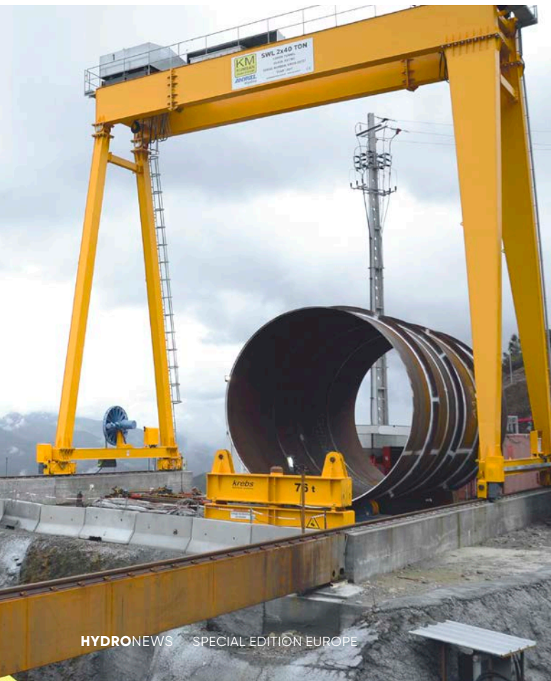
On site installation work Gouvães, Tâmega River
