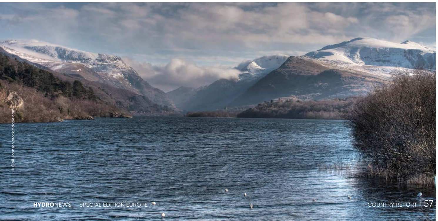
Dinorwig Pumped Storage Plant, Wales
