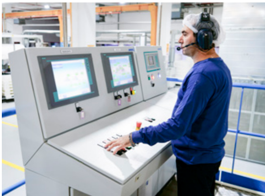
Monitoring system for process supervision
