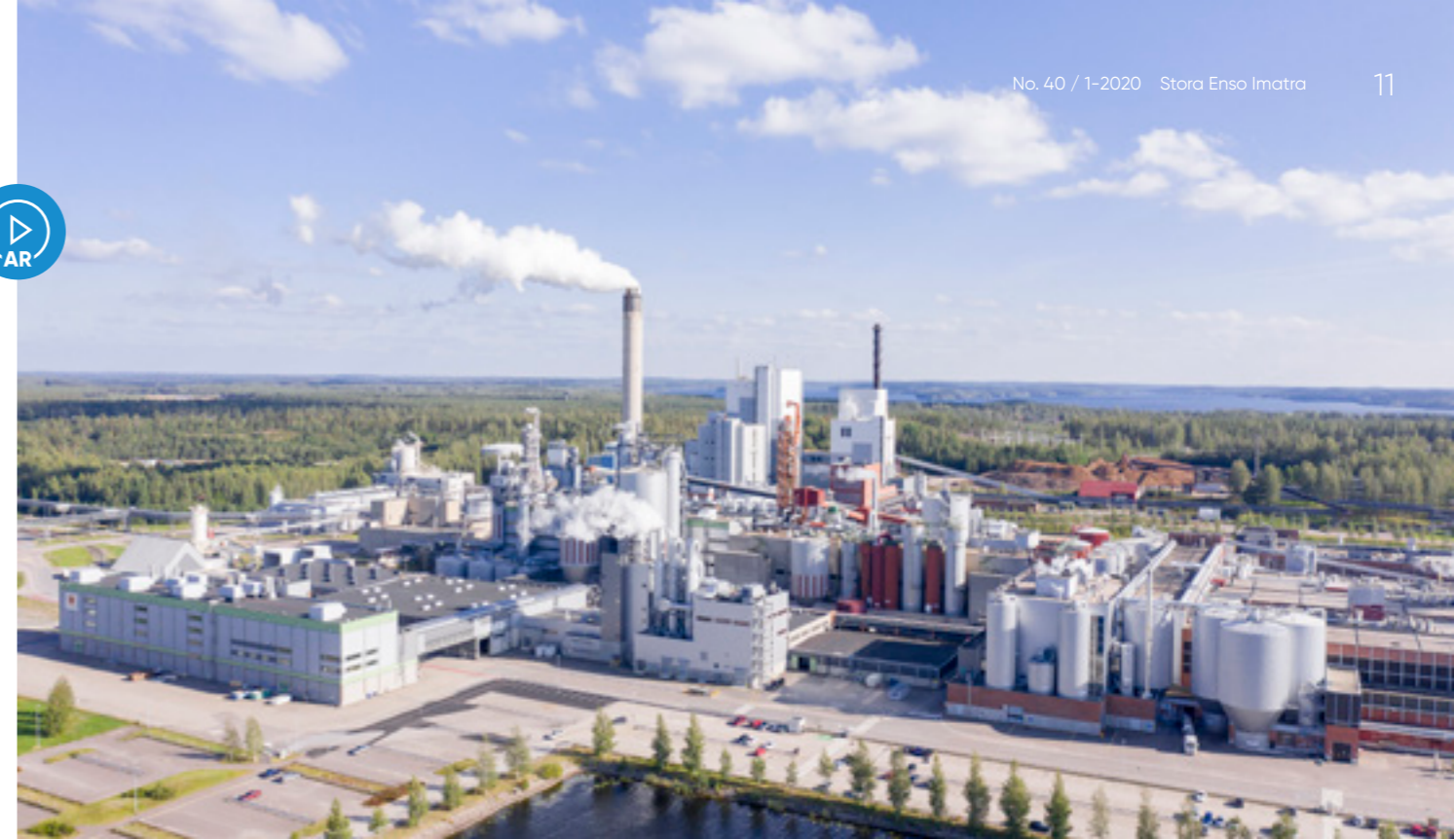
Stora Enso Imatra and ANDRITZ together developed how to locate the Flash Drying plant in an efficient space in the mill. The new Flash Drying Line was fitted into the overall layout.
