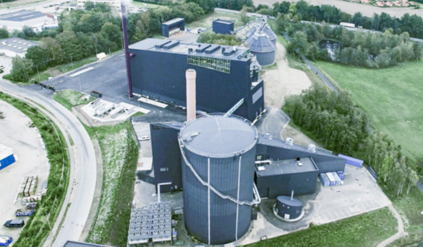
ANDRITZ's scope of supply included the boiler island, from fuel silos to boiler outlet, based on its Ecofluid BFB boiler design.
