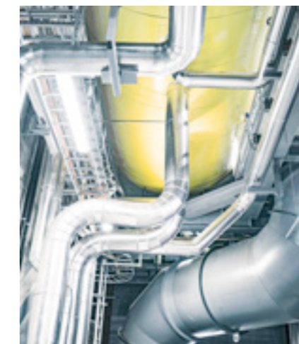
The plant is now fully operational and ready for its first winter of operation.
