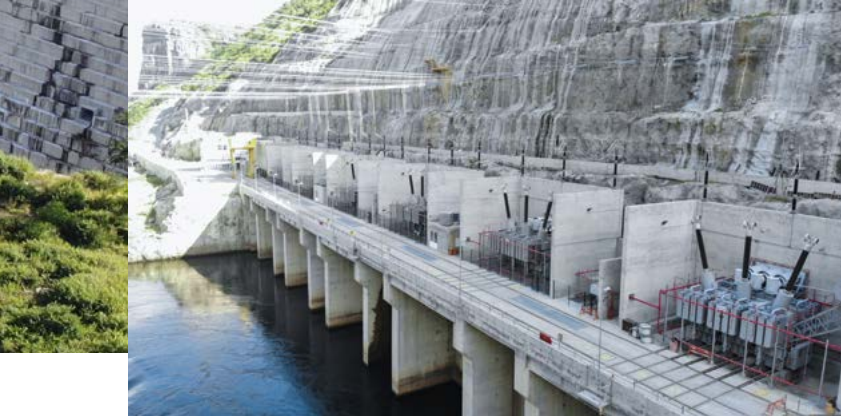
Laúca increases not only the available electrical power, it is also the backbone of modern grid regulation in Angola.
