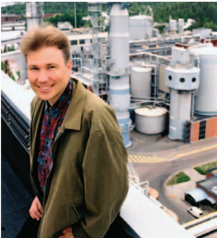
Above: Auvo Kettunen, Development Manager for Cooking Processes at Andritz. Right: The softwood digester (left) rebuilt by Andritz produces 200,000 t/a bleached softwood pulp. It utilizes Downflow Lo-Solids® Cooking and Enhanced Alkali Profile Cooking (EAPC) to improve pulp strength and yield. The new 1000 t/d Andritz digester (right) with Lo-Level® Feed and Lo-Solids® Cooking has performed with 100% availability.
