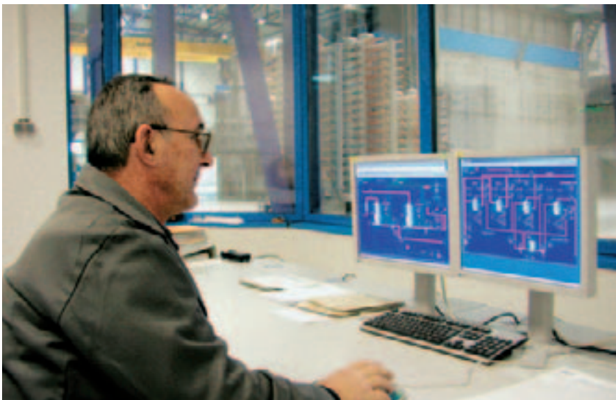
Only one operator is needed to run the entire DIP facility. The Andritz cleaner plant can be seen through the control room window in the background.
