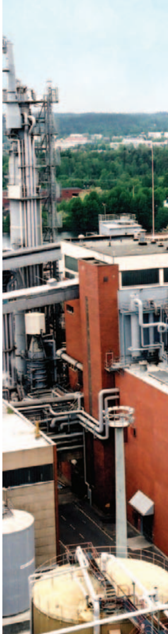
Above: Auvo Kettunen, Development Manager for Cooking Processes at Andritz. Right: The softwood digester (left) rebuilt by Andritz produces 200,000 t/a bleached softwood pulp. It utilizes Downflow Lo-Solids® Cooking and Enhanced Alkali Profile Cooking (EAPC) to improve pulp strength and yield. The new 1000 t/d Andritz digester (right) with Lo-Level® Feed and Lo-Solids® Cooking has performed with 100% availability.
