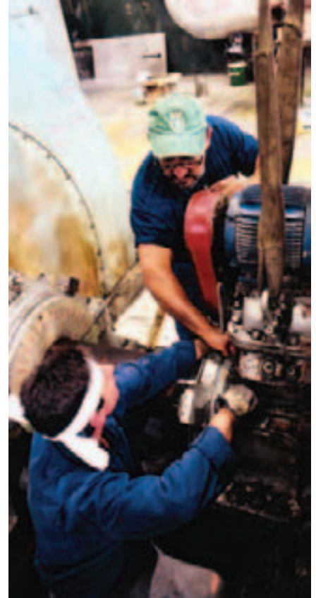
ASIP workers replace the bearings on a back-up turbine generator at the mill.
